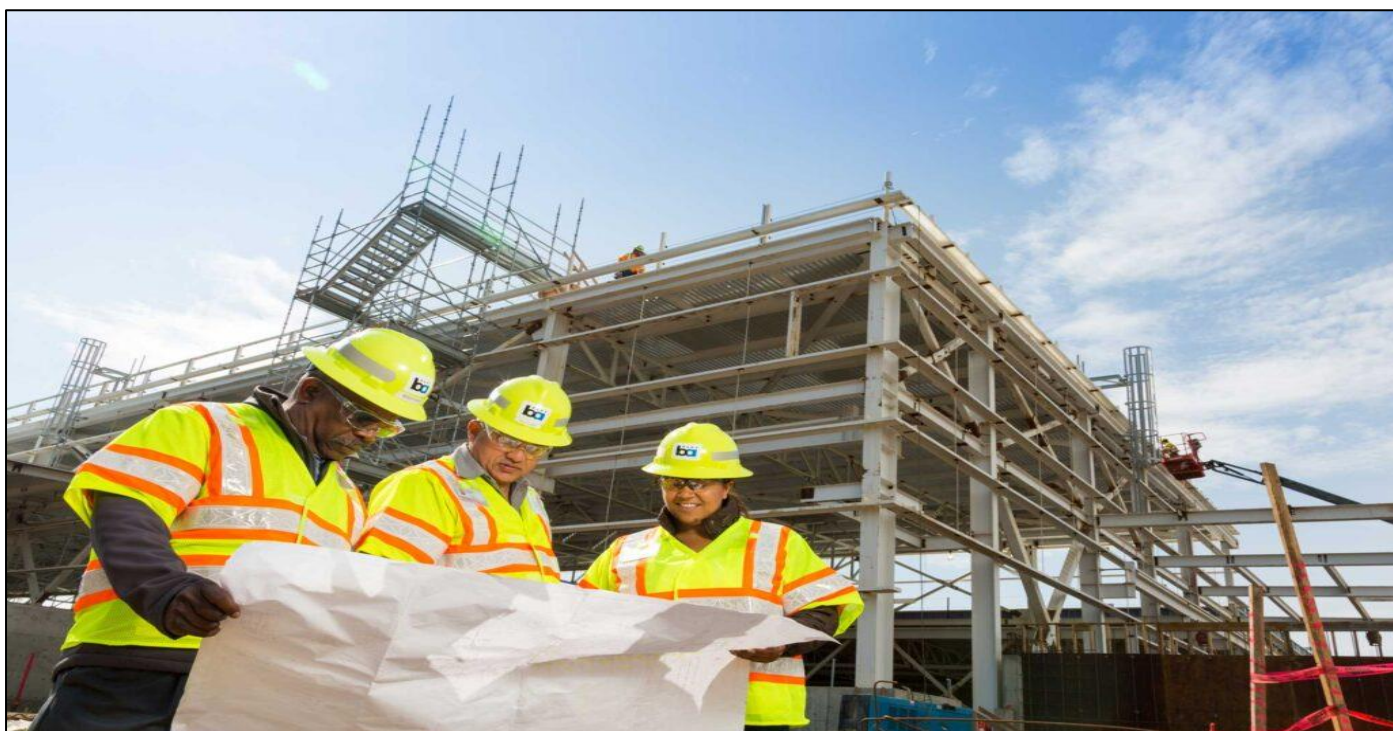
Fig 1 Collaborative on-Site Planning in Modern Construction Management (The Architecture Designs, 2023).
