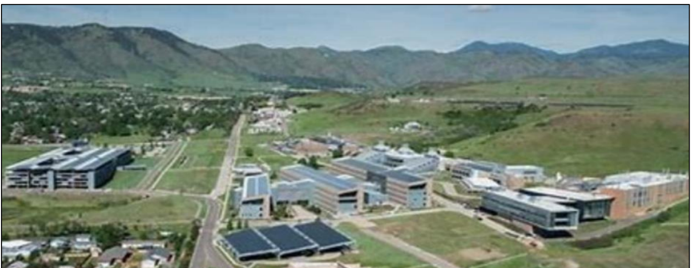
Fig 2 The Site of the National Renewable Energy Laboratory (NREL), USA Source: Arch Daily (2010)
