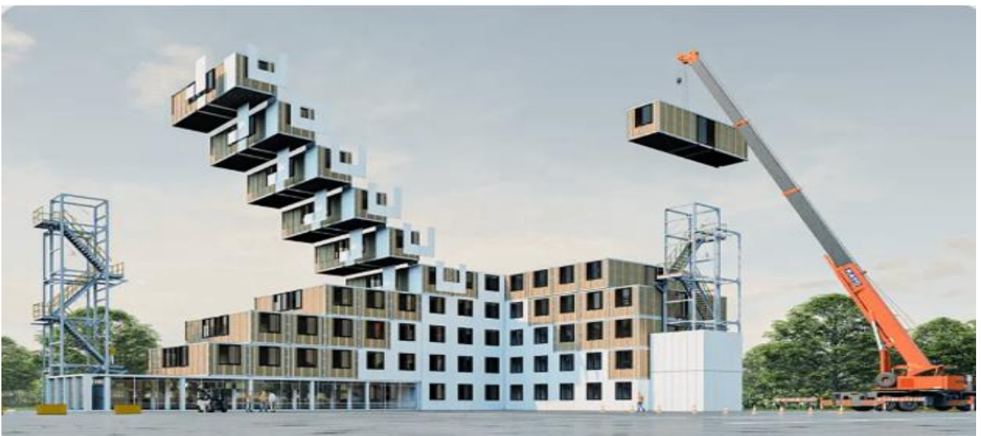
Fig 2 Volumetric (3D) Modular Construction Source: Research Gate, 2015
