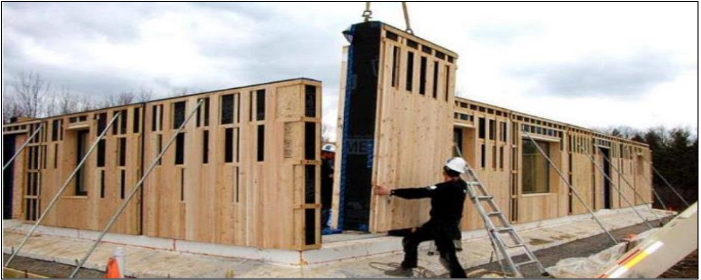
Fig 1 Panelized (2D) Modular Construction Source: Google, 2018
