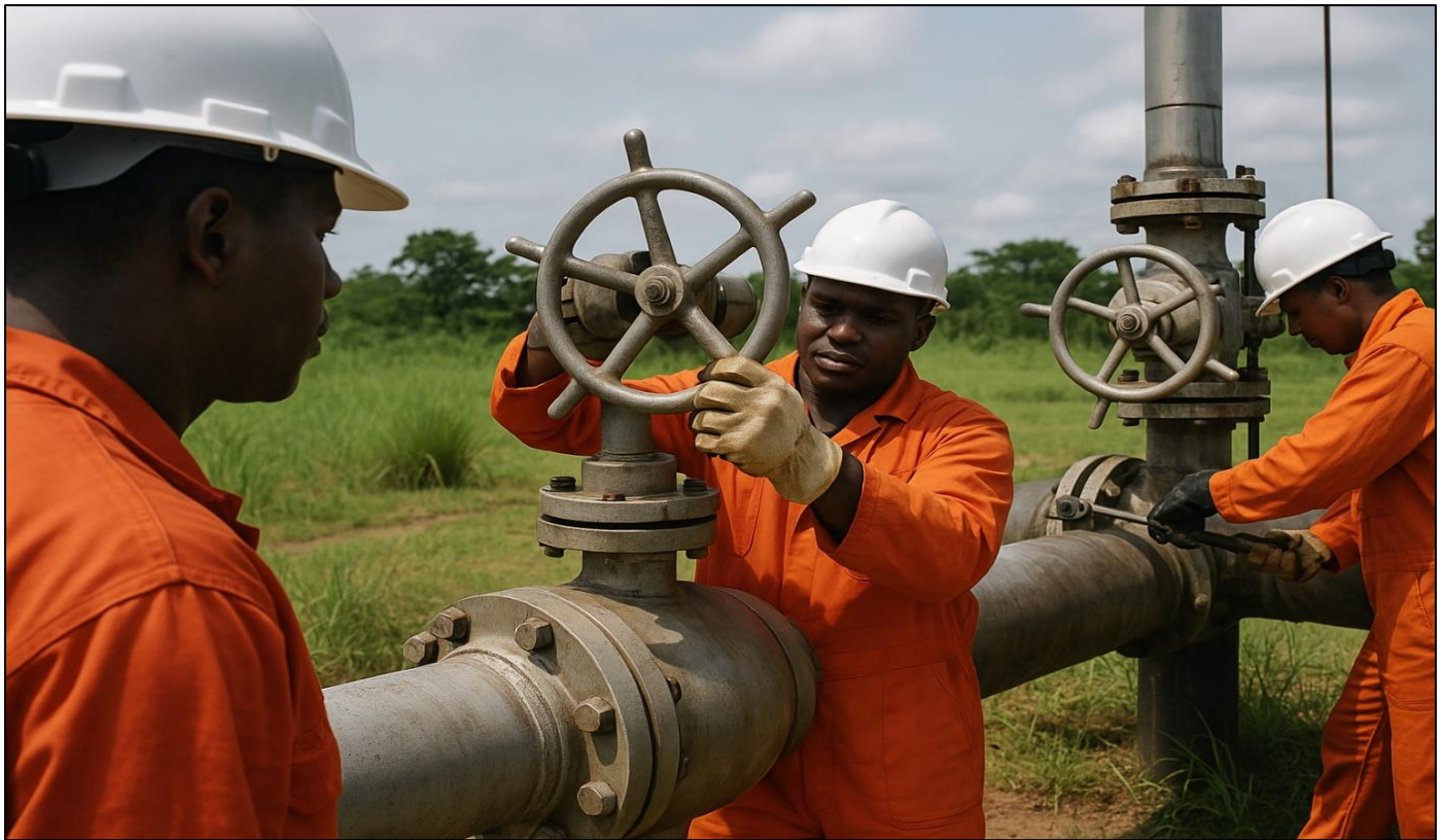
Fig 1 Field Maintenance Activity in Gas Transmission Operations
