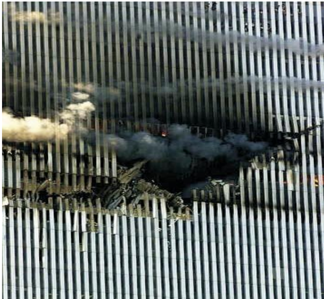
Fig 1:- A "clean" cut driven into the North Tower's facade by the wings of a Boeing 767
